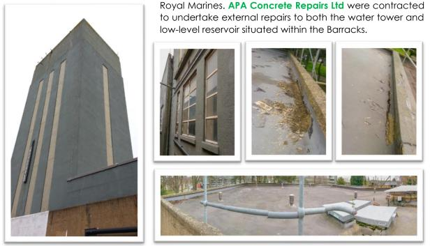
**The solution:** Visual and hammer tap surveys were first undertaken in order identify the necessary repairs. Areas of defective concrete were then broken out, the substrate and existing reinforcement were prepared, and the repair areas were reinstated using proprietary
